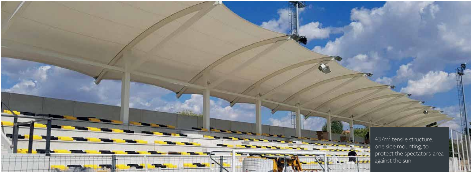
5 hypar membranes, made of 'mesh' fabric Valmex TF, which combines sun-protection and perfect view towards the sky
